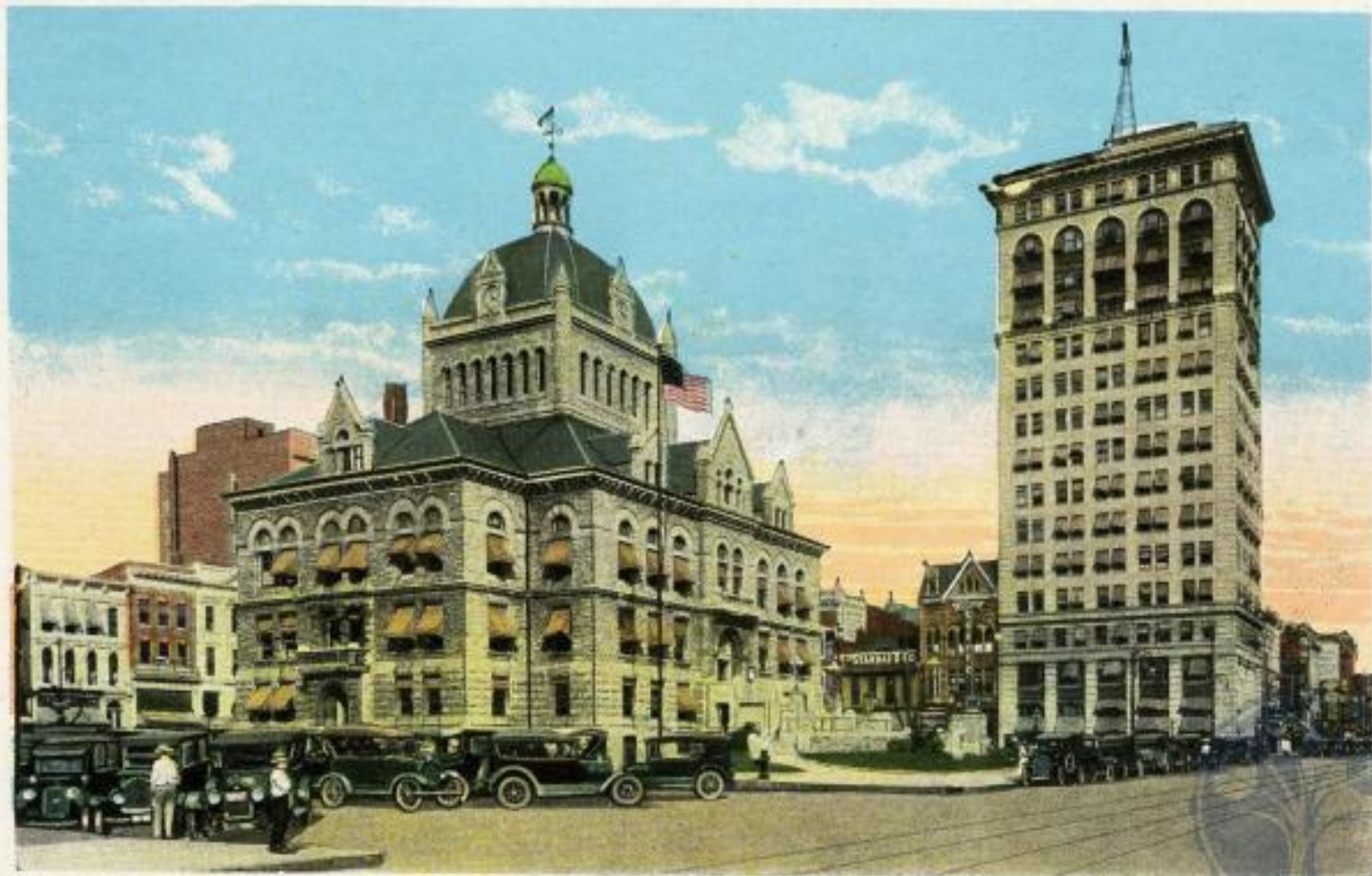
Fayette County Court House.
