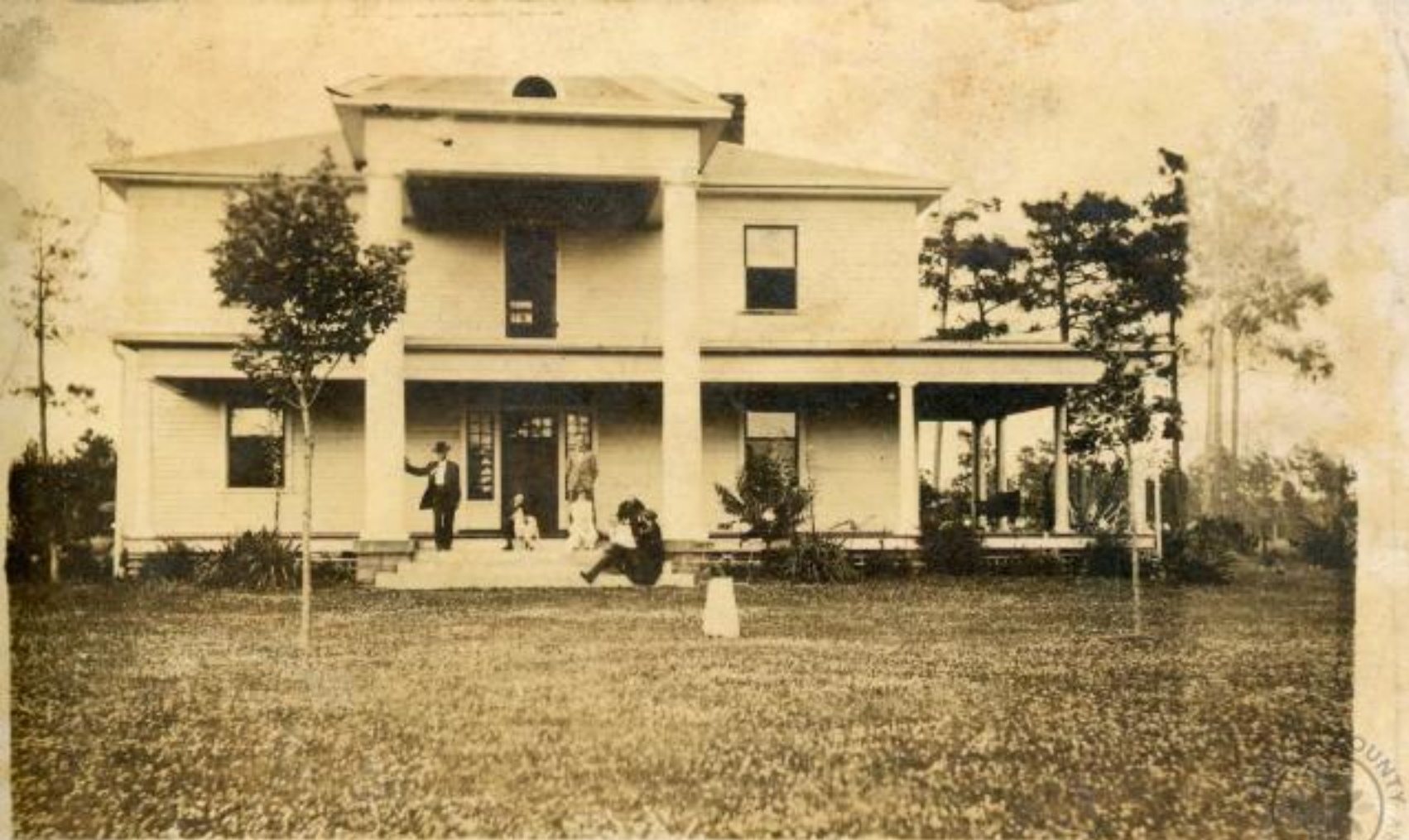
Kodak failed to catch all the roof
