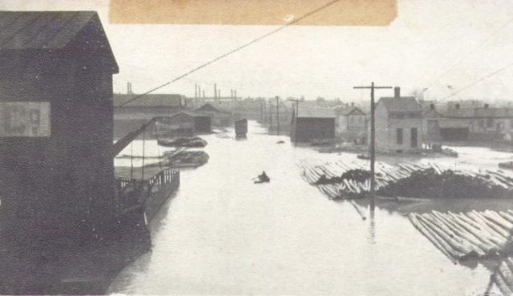
A scene from 11 th Street Bridge--Newport, Ky. Flood, January 1907.
